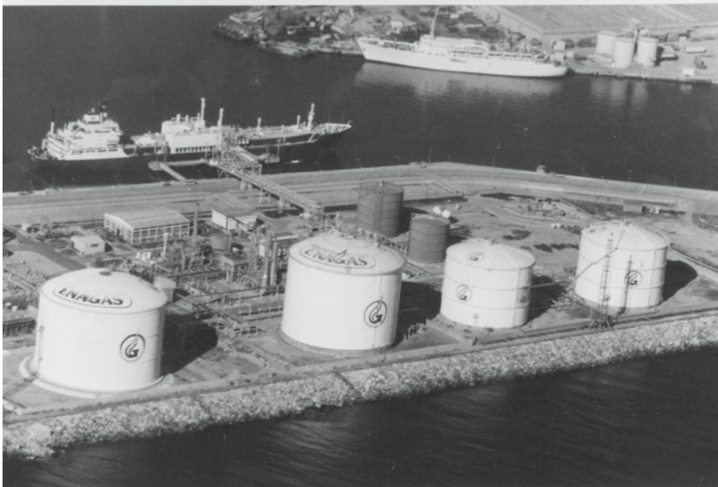
(2) 40,000-m 3 LNG Tanks With Prestressed Concrete Inner Wall 1969
